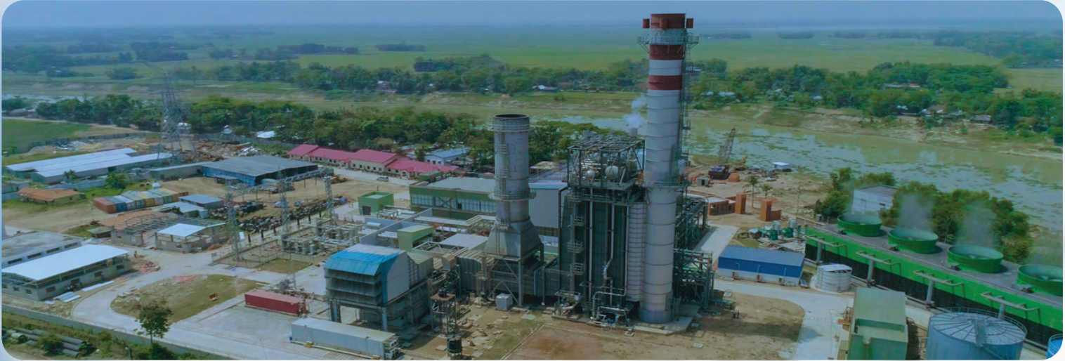
EPC Project: KPCL 163 MW Combined Cycle Power Plant. Transmission Line, 230/11KV GIS Substation.
