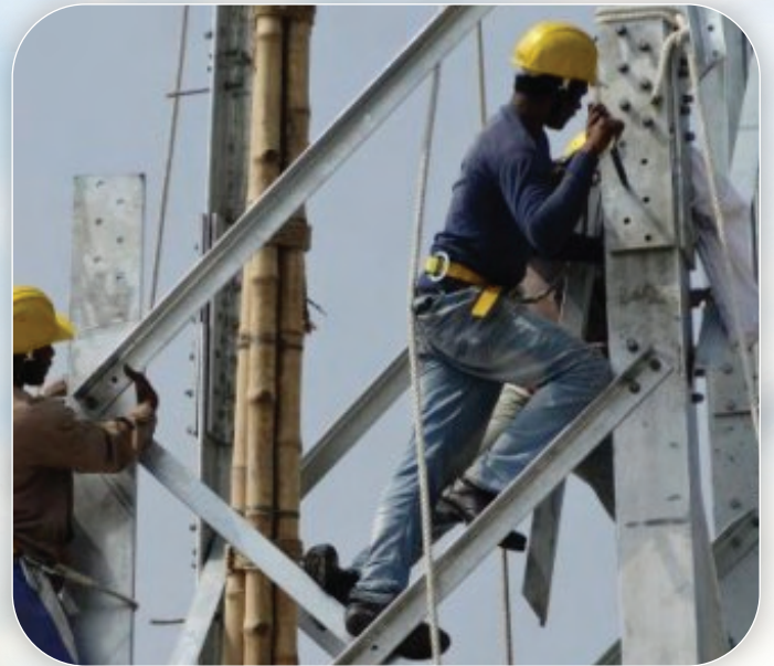
Tower Erection Work
