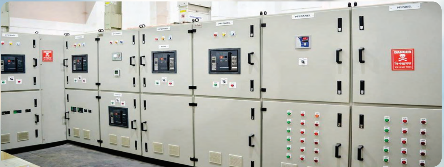
Epillion Washing Limited: Supply, Installation, Testing & Commissioning of 5 MVA, 33/11KV Electrical Substation & 2.5MVA 11KV/.415KV Electrical Substation
