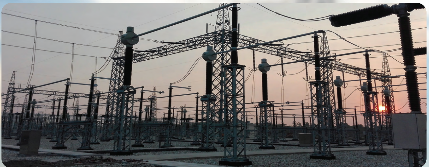
Project: Erection, Testing and Commissioning PGCB 230/132kV Substation, Barisal
