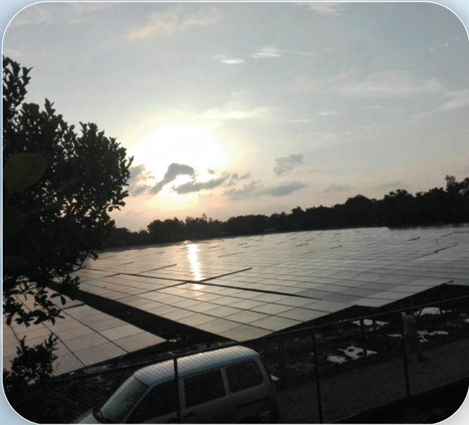
Solar Power Plant Project: Electrical Power Evacuation for 3MW Solar Power Plant at Energreen Sarishabari.
