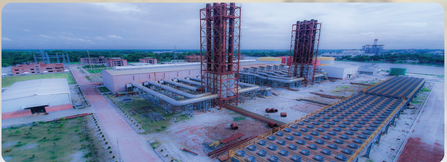
EPC Project: EBoP 200MW HFO Power Plant with 132kV GIS Substation at Desh Energy, Chandpur
