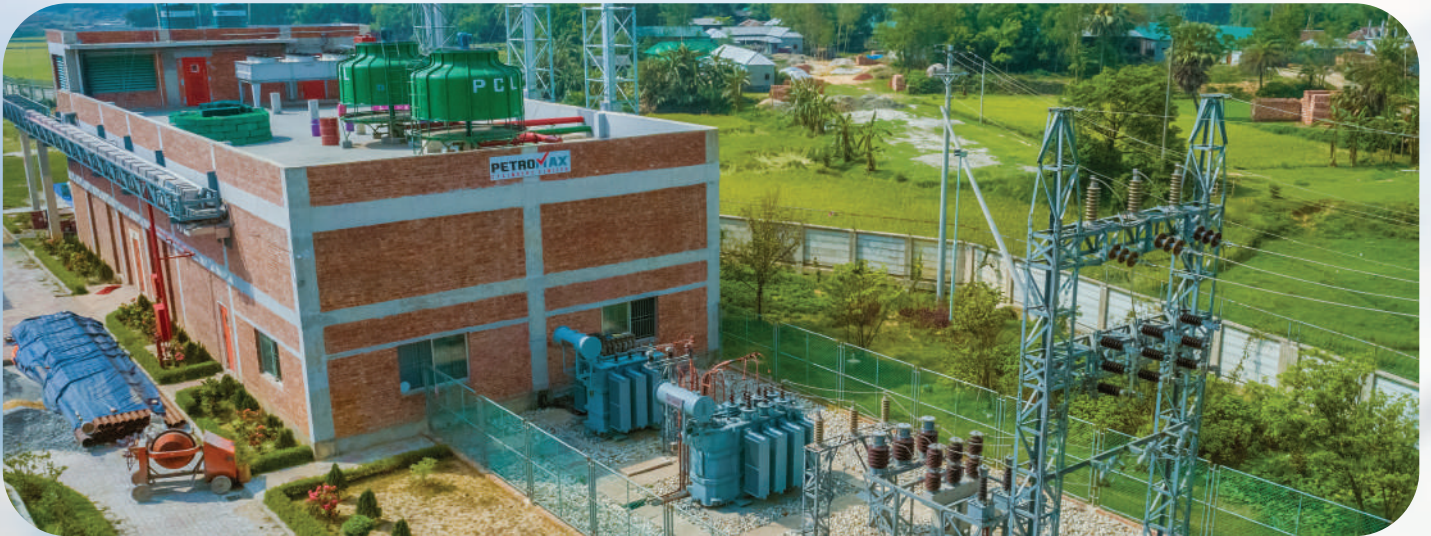
Petromax Cylinders limited: Supply, Installation, Testing & Commissioning of 4 MVA, 33/11kV with 4MVA 11kV/.415kV Electrical Substation with 1000KW GAS Generator Synchronization with REB Including Central Load Monitoring System.
