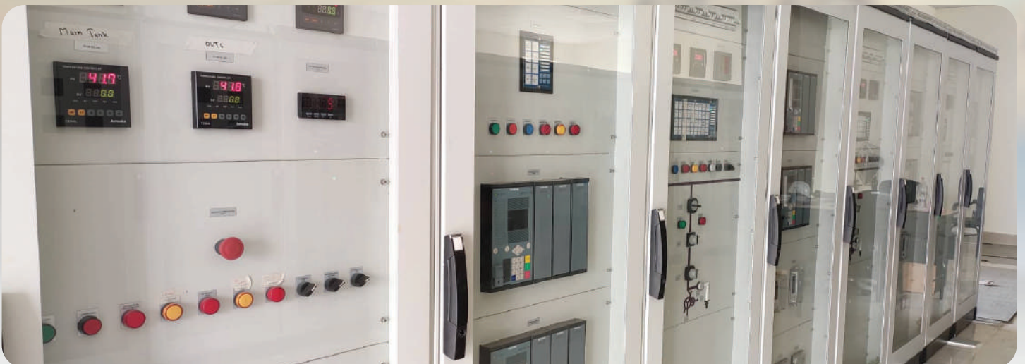
EPC Project: 400KV Control, Relay and Protection Panel at PGCB 400KV Payra Substation (Gopalganj)
