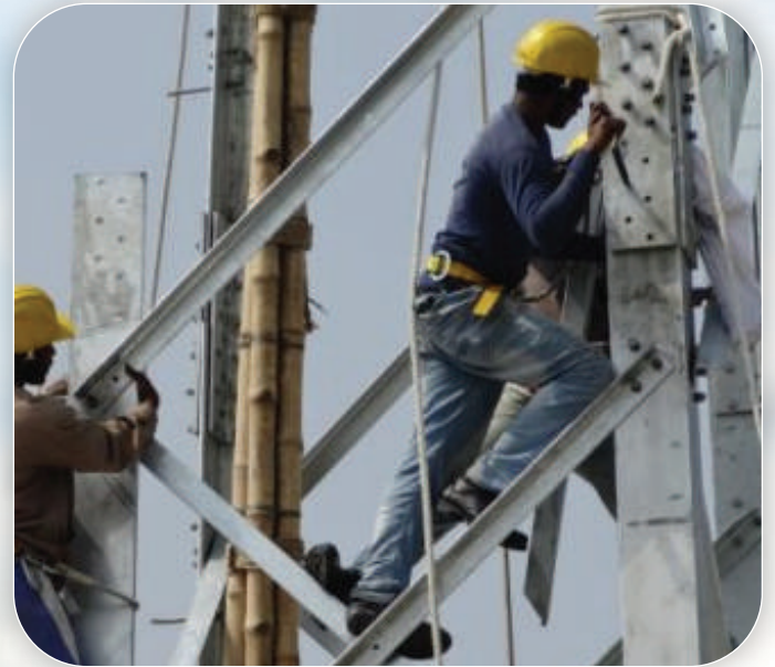
Tower Erection Work
